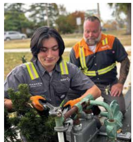
Chad Bailey works to replace a home gas meter while his Spire mentor, Eric Jobe, provides onsite guidance and training.
